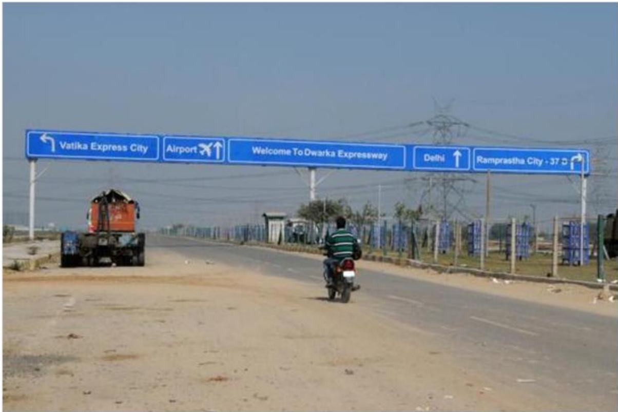
The elevated road will start from Gurgaon-Delhi border and end near the Basai railway overbridge in Sector 100. (HT File)
